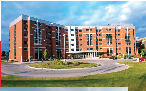
Merlin House Residence
